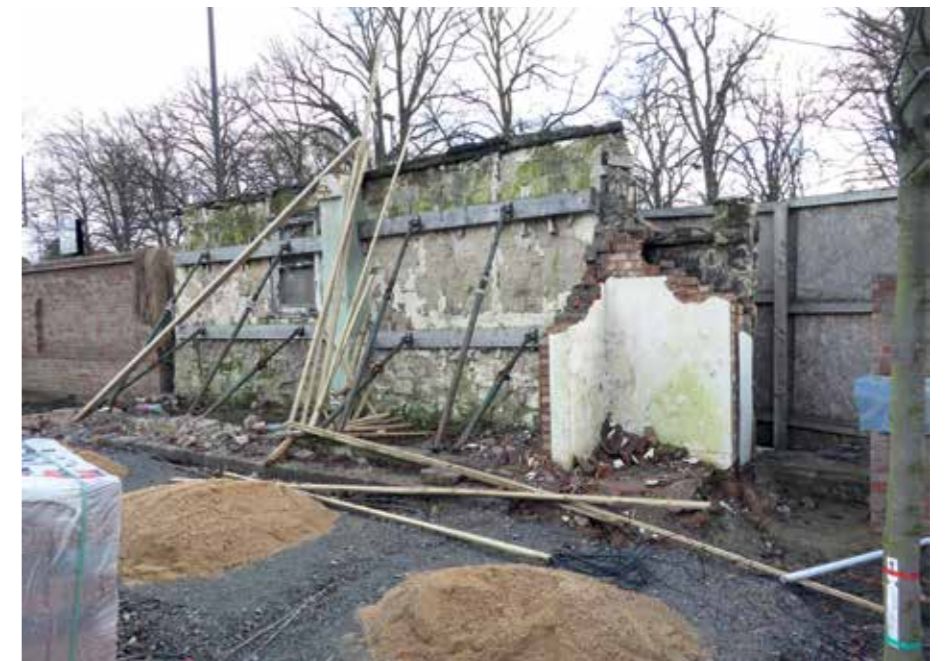
The Clunch Wall Panel, temporarily supported and awaiting repair
